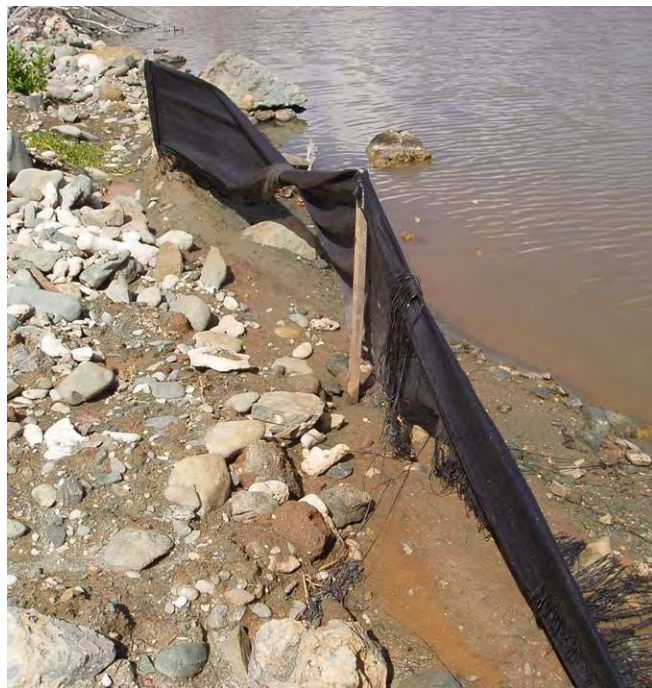
Improperly maintained sediment fence along salt pond shore.
